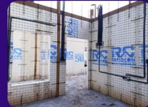
How to do the concealed electrical-plumbing work on EPS panel
