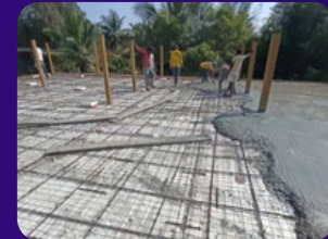
Slab reinforcement and concrete work
