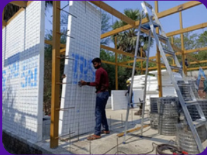
How to Install EPS wall panels on a structure or non-structure building
