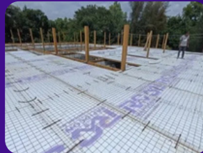
Installation of EPS panel slab
